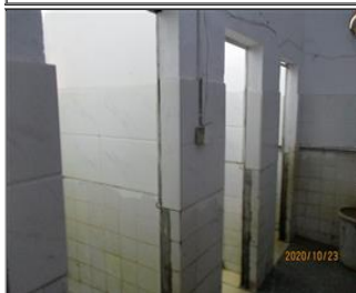
Photo of the sanitary facilities Toilet.JPG
