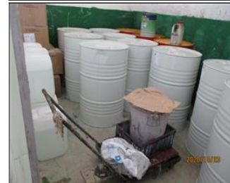
Photo of non-conformity NC 7.7 No secondary container.JPG
