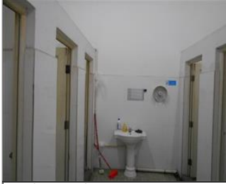
Photo of the sanitary facilities Toilets.JPG
