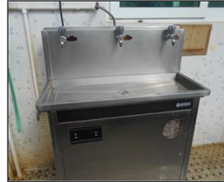
Photo of the inside of the main production hall Drinkable water supply.JPG
