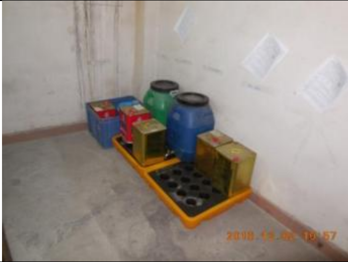
Chemicals were stored with secondary containment.
