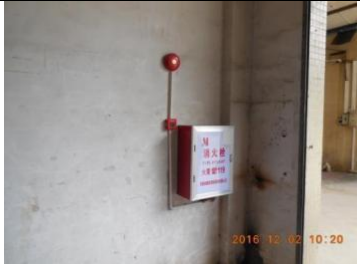
Fire alarm and fire hydrant
