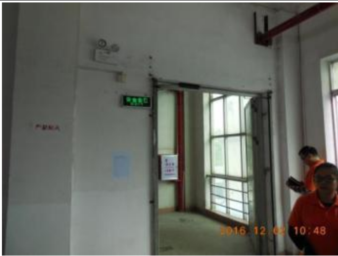
Exit sign and emergency lighting
