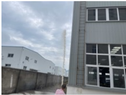
Fire Hydrant testing
