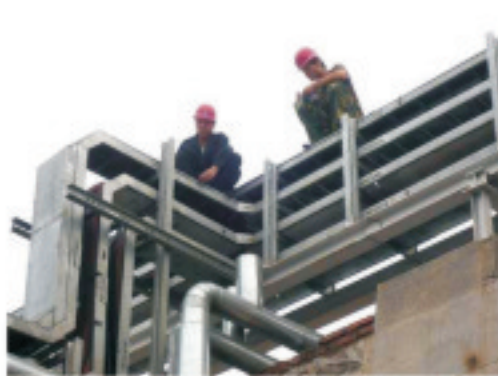
Yulong FRP Cable Bridge used for the railway project
