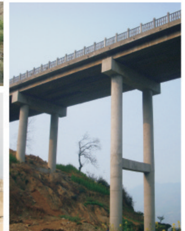
Yulong FRP rib materials used for Bridge construction
