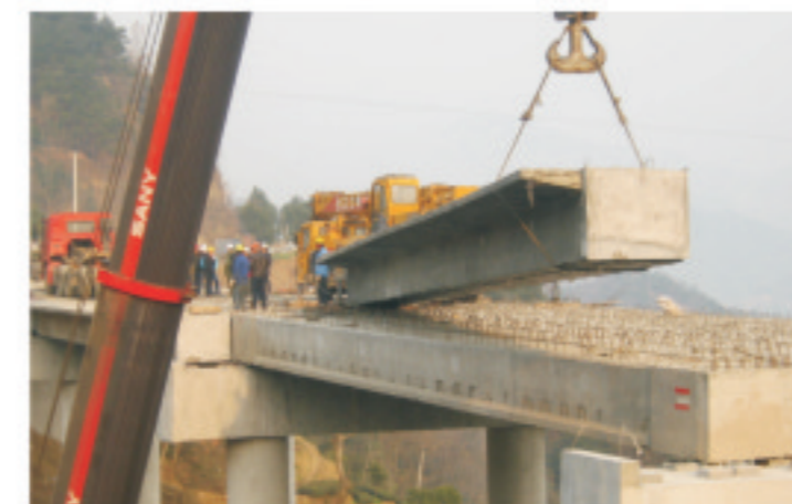
Yulong FRP rib materials in the site construction
