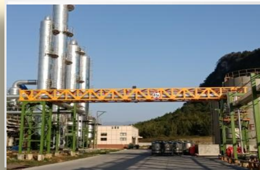
DMFa Recovery Tower
