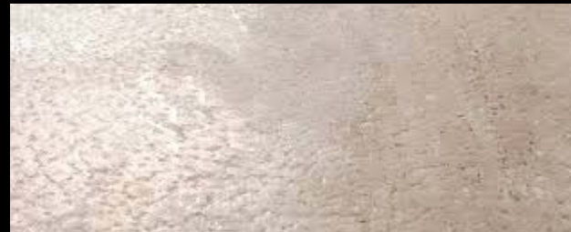
Acid Finish Slab
