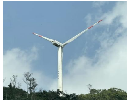
Wind Power Equipment
