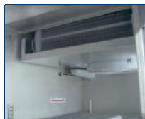
顶部安装蒸发器 top mounted evaporator
