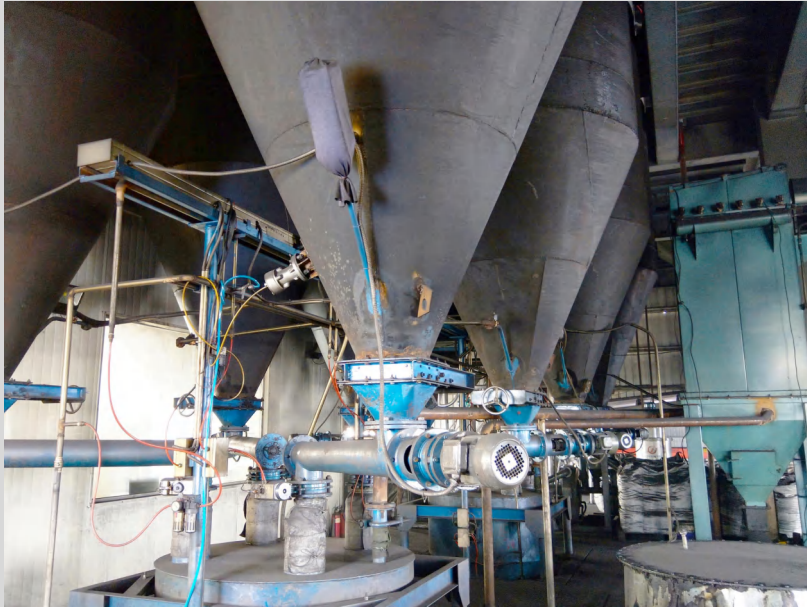
Raw material batching & mixing
