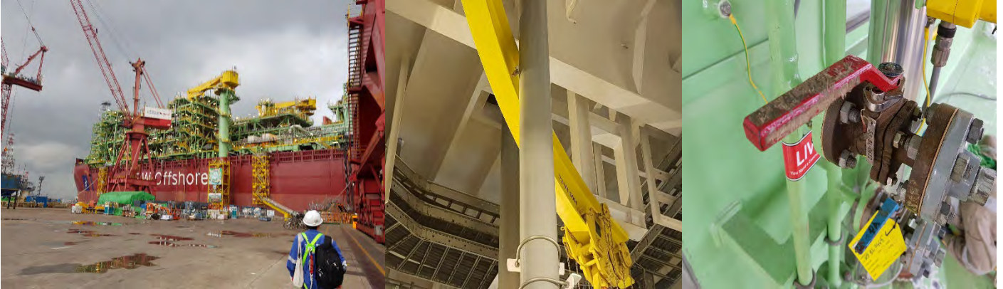
BWO H.5003 Catcher FPSO Singapore Keppel Commissioning
